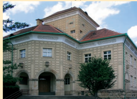
The building of Hus' School in Krušovice
